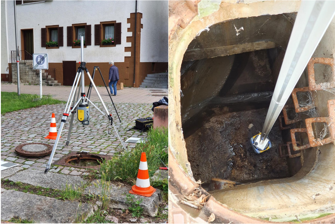
Figure 6: Inverted scans leveled with survey grade accuracy. Photo from Karsten Braun; Dipl. Ing. | Vertriebsingenieur; Beim Erlenwäldchen 8 | D-71522 Backnang
