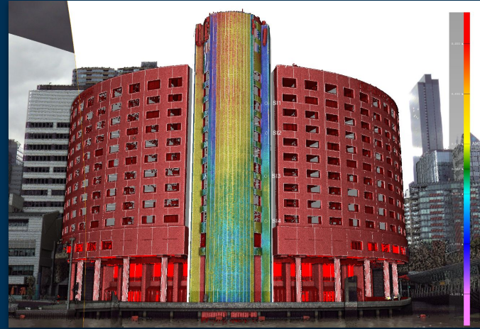
PERFORM SCAN INSPECTIONS BETWEEN OBJECTS IN TBC
