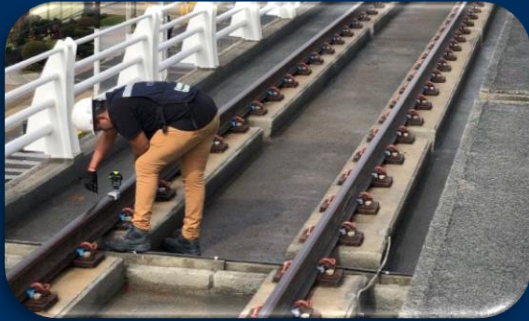
Survey rail coordinates with rail shoe and track bar
